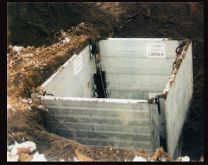
ALUMINUM SHORING ON SITE
